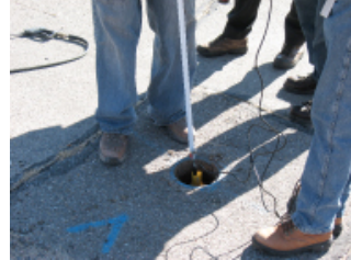
Deploying an acoustic leak detection logger
